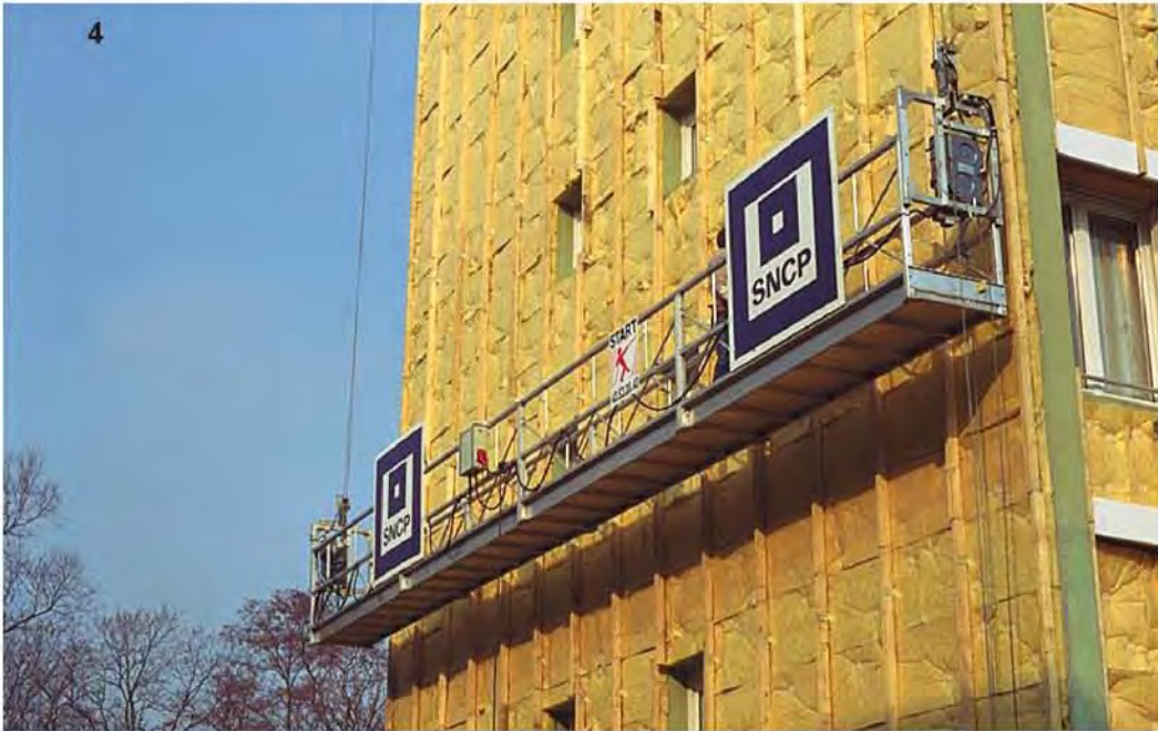
4 - ALTA suspended cradles are made up of modular sections of 2 m and 3 m and can be assembled to reach the length required. These sections can even be assembled to make platforms with several decks. Fitted with TIRAK powered hoists.
