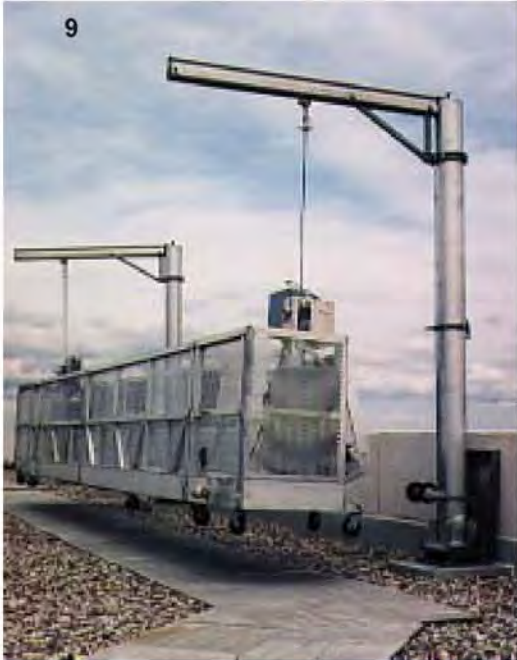
9 - SSL-type removable davits may be turned into the required position so that the different sections of the facade can be reached.
