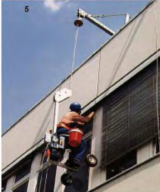
5 - The powered one-man lift SOLSIT is a particularly lightweight and economic solution for urgent repairs. Whether for ALTA platforms or for the SOLSIT, we recommend mobile roof rigs or parapet clamps. Sometimes an original solution is called for; we can do that.
