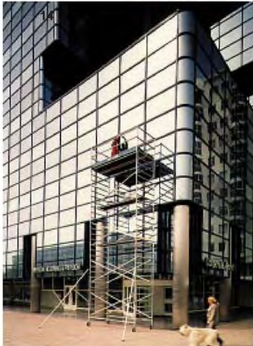
IDEALSCAF mobile aluminium scaffolding tower • max. height of the floor panel: 20.2 m • maximum load: 675 kg
