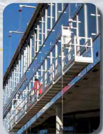
ALTA suspended platform from 2 Portafix jibs, Luxembourg (L)
