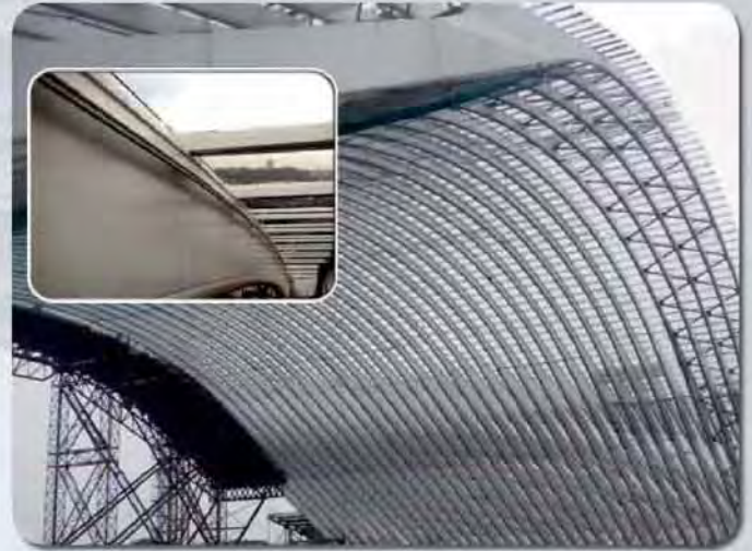
I-SCAF, TGV railway station, Liege (B)
