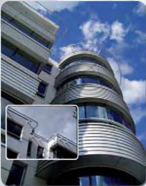
RAILSCAF with SOLO platform, St. Denis (F)
