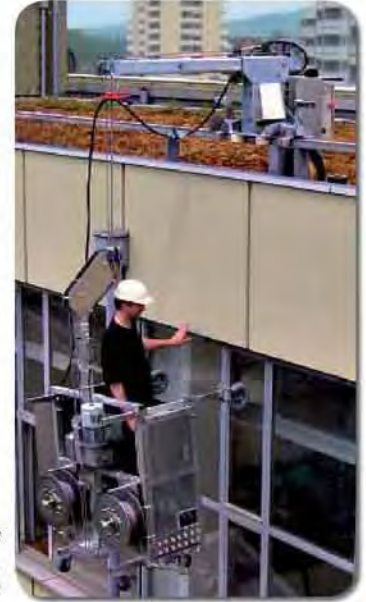
Powered Davits with SOLO platform, Basel (CH)
