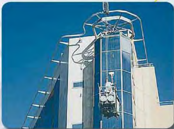
Suspended platform from traversing trolley on monorail, Morocco (M)
