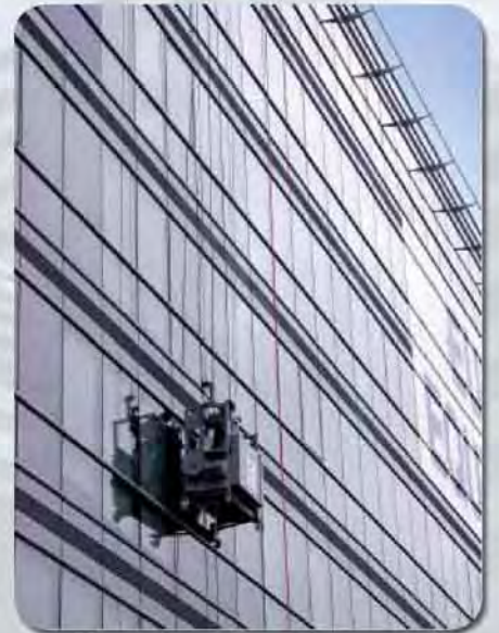
RAILSCAF with ALTA platform, Paris (F)
