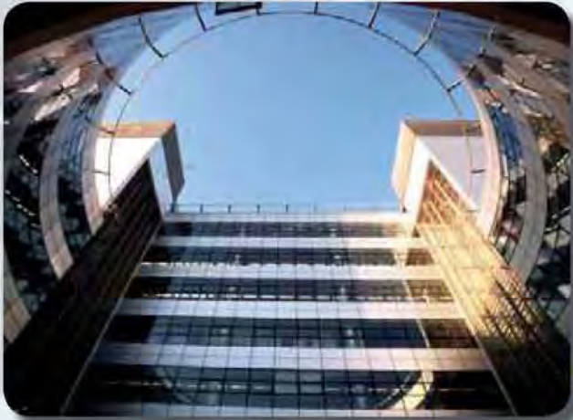
Horizontal RAILSCEF, Brussels (B)
