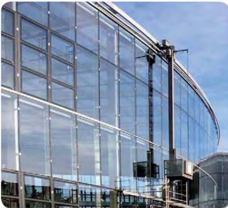
Polelift, Geneva (CH)
