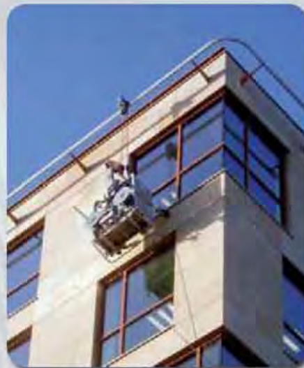
RAILSCAF with SOLO platform, Paris (F)
