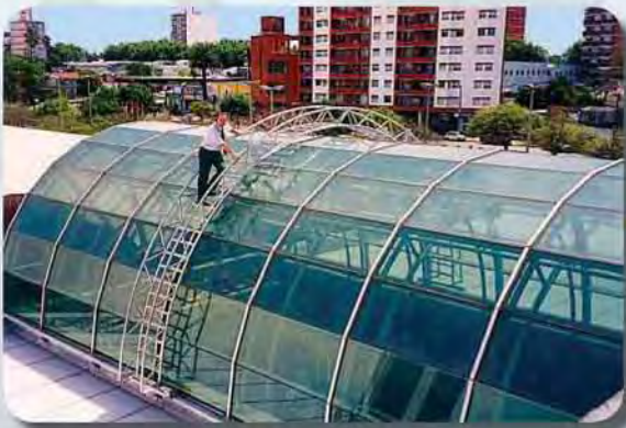
Ladder for external maintenance of glazed surfaces, Paris (F)
