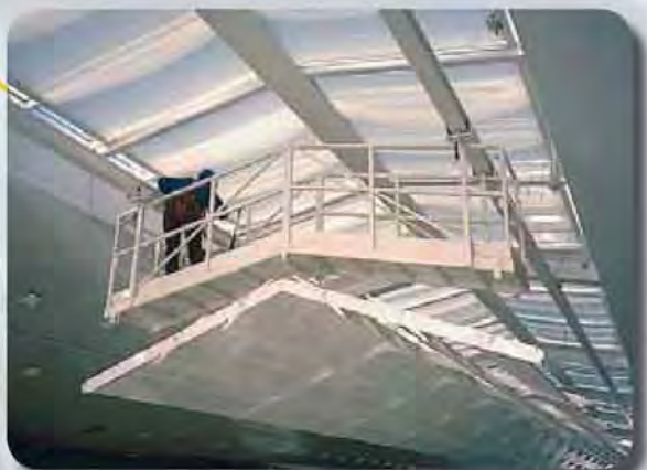
Travelling gantry for internal maintenance of glazed surfaces, Dublin (IRL)
