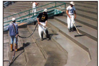
Concrete resurfacing.
