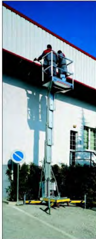
2 operators for erection work
